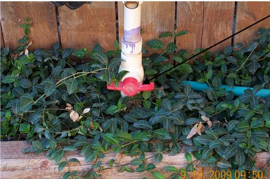
**IN THE SPRING**, when notice is given that the water will be turned on, turn your valve to this position so that the main system can be pressurized. After the system is pressurized, you may turn your valve to the open position for watering.
